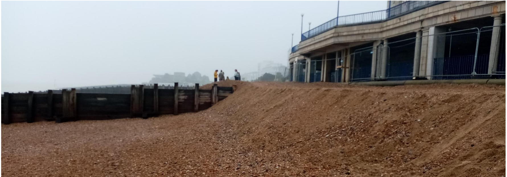
Figure 4: The Bandstand beach after reprofiling work undertaken on 1st March 2022. Photo G. Caira. There appears to be more sand than shingle in the newly formed beach head. This mix of sand and shingle does not provide much protection and is easily washed away by storm waves.
