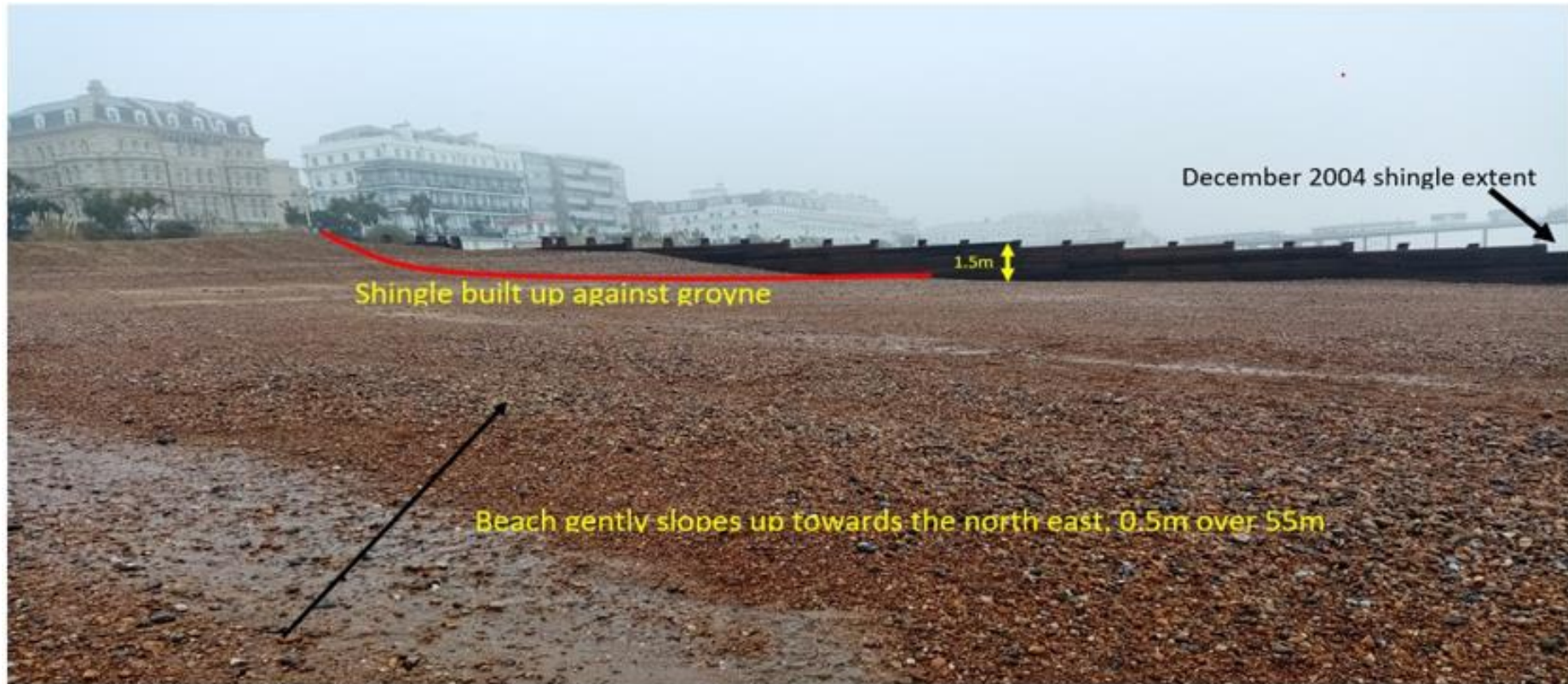
Figure 3: Northeastern side of the beach. The beach gently slopes up from the SW to NE laterally across the beach. The red lines follow the approximate trend of the deposit against the opposite groyne. Taken on 1 st March 2022 after the three named storms had eroded and reprofiled the beach.
