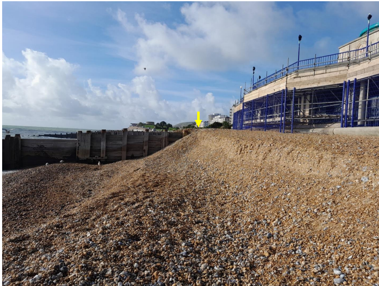
Figure 2: The Bandstand beach on 22 nd Oct 2022. The beach has been recharged following the February storms and then eroded back around 17m during the summer and autumn. Photo G. Cairra.
