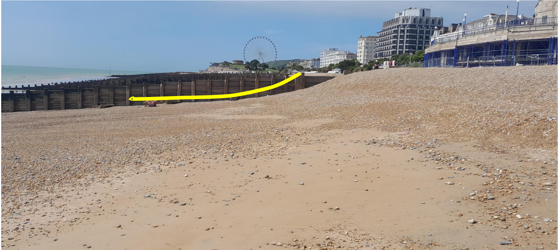
Figure 5: Bandstand beach on 10 th July following long Spring tides, between the 4 th and 6 th July, combined with 1m swell waves impacting from the south west. This relatively benign set of marime conditions has stripped back a significant amount of the newly recharged beach. Photo G. Caira.
