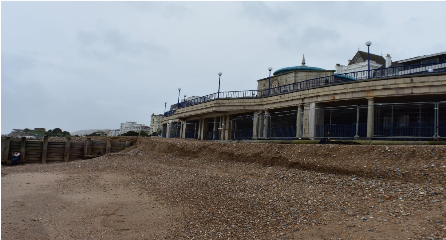
Figure 2: The beach after storm Dudley and initial impact of storm waves. There is a significant sand content in the beach deposit mixed with small round pebbles that has very likely contributed to the apparent acceleration in erosion since 2018. Photo G. Caira.
