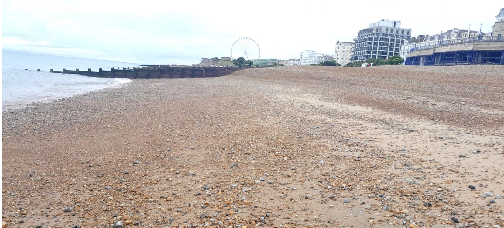
Figure 4: The Bandstand beach on 29th June 2023. Using the beach loss model from the survey conducted in February 2022, the beach has been recharged with around 1000 m 3 of unsuitable ballast. Which at previous costs of £15 per m 3 equates to another £16,500 on just one of many beaches. Photo G. Cairn.
