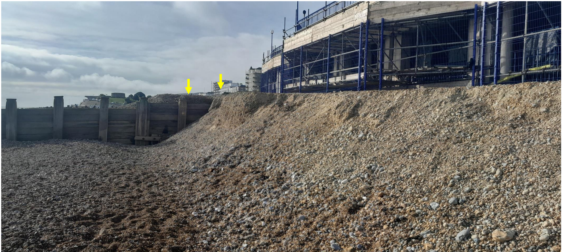
Figure 3: The Bandstand beach on 2 nd March 2023. The yellow arrows indicate the distance the shingle sand mix has eroded back another 1.5 m over the winter. Photo G. Cairn.
