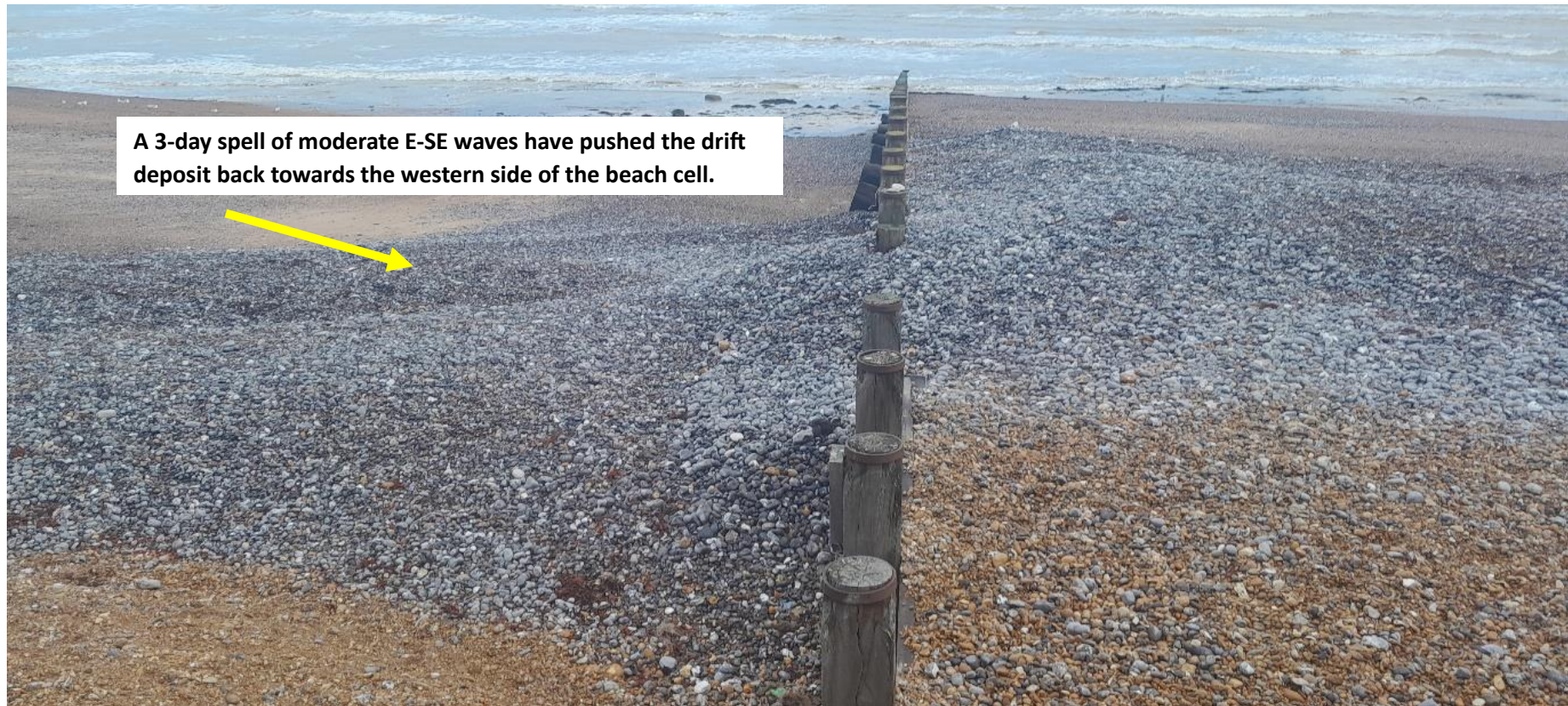
Figure 4: Grey cobbles overtopping the eastern groyne of a beach cell. The cobbles on the eastern side (left) have been subjected to a short period of waves impacting from a E-SE direction, this has reversed the direction of prevailing drift.
