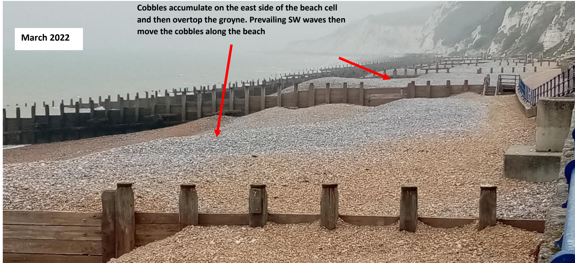
Figure 14: The beach above is becoming stable as further drifted cobbles are washed over the groyne on the western side of the beach cell. The cliffing apparent along this beach in October 2018 (see Figure 10) has been eliminated as the sand is washed out and larger grey angular clasts are introduced.
