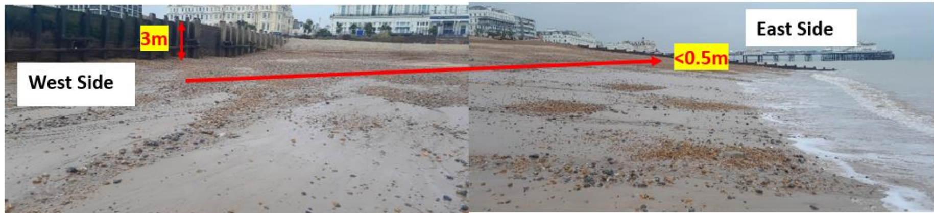
Figure 5: The anthropogenic sediments, a chaotic mix of sand gravel and occasional cobble, are easily drawn down the beach and then pushed up against the eastern groyne by prevailing SW waves. The sediment level along the west side of the beach cell is in excess of 3m below the top of the groyne structure. The sediments slope up towards the east side to within 0.5m of the top of the groyne. Considerable stress is applied to the groyne by the weight of ballast and the smaller shingle will overtop the groyne further down than the larger grey cobbles.
