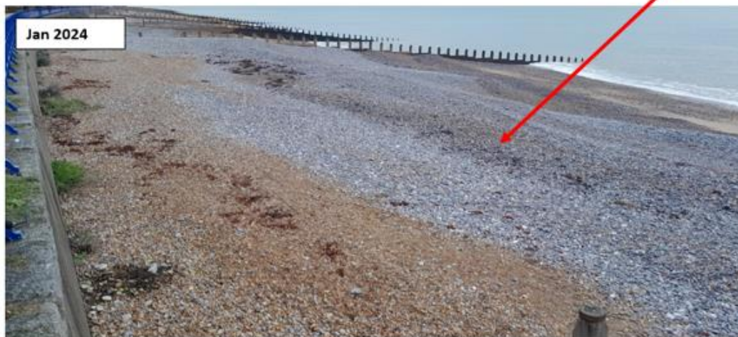
Figure 13: In under two years sufficient cobbles have drifted onto the beach and stabilised it. Only a relatively thin veneer 5m wide stretching across the entire beach is required to prevent erosion. There is actually a surfeit of cobbles on this beach with the excess above minimum load deposited below the HW berm. Cuspate features have been formed within the lower section.
