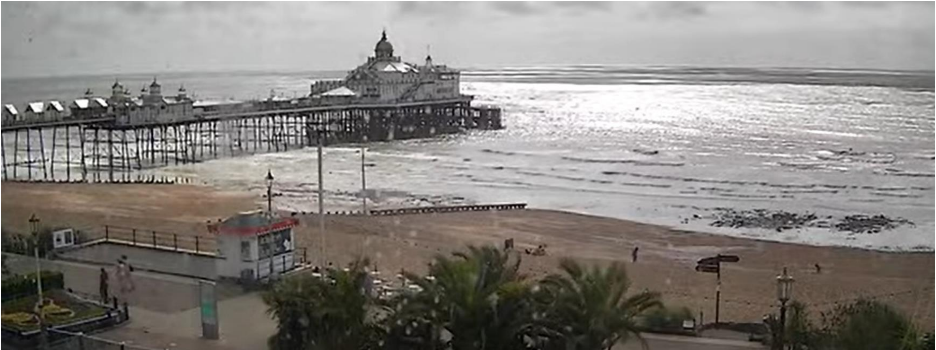
Figure 10: Between 2 nd and 23 rd July 2023 a significant amount of sand and shingle has drifted down and across the beach. Compare the exposure of the wooden groyne in the center of the images with that in Figure 9, above. Image from beach camera at the end of Terminus Road.
