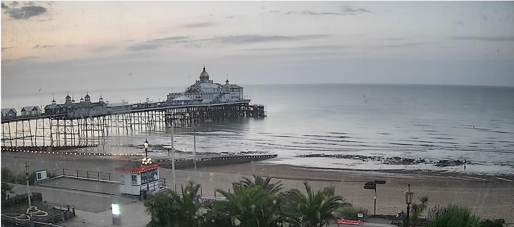
Figure 9: Between 21 st April 2023 and 2 nd July 2023 a significant amount of sand and possibly small shingle has covered some of the Gault previously exposed on 21 st April 2023. Image from beach camera at the end of Terminus Road.
