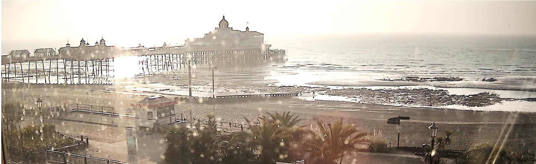
Figure 8. In the 13 months between the dates of the two photos the surficial cover of Sand has been eroded away exposing Gault. The groyne is also significantly more exposed compared to February 2022. Image from beach camera at the end of Terminus Road.
